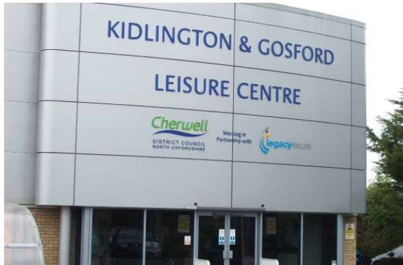
Figure 2.20 Gosford - leisure centre
